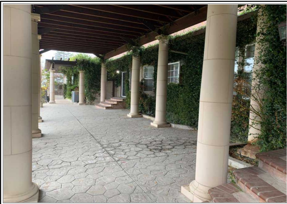
REAR OF SUBJECT PROPERTY
