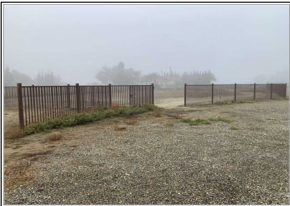
Partial view of extensive wrought iron fencing
