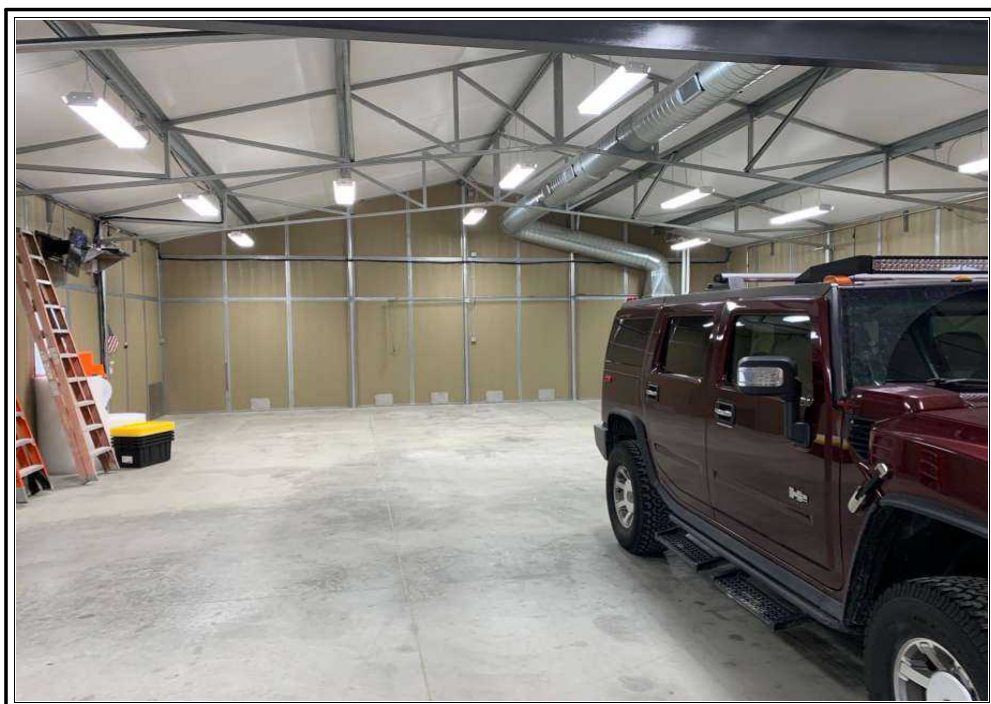
Interior view of shop 2
