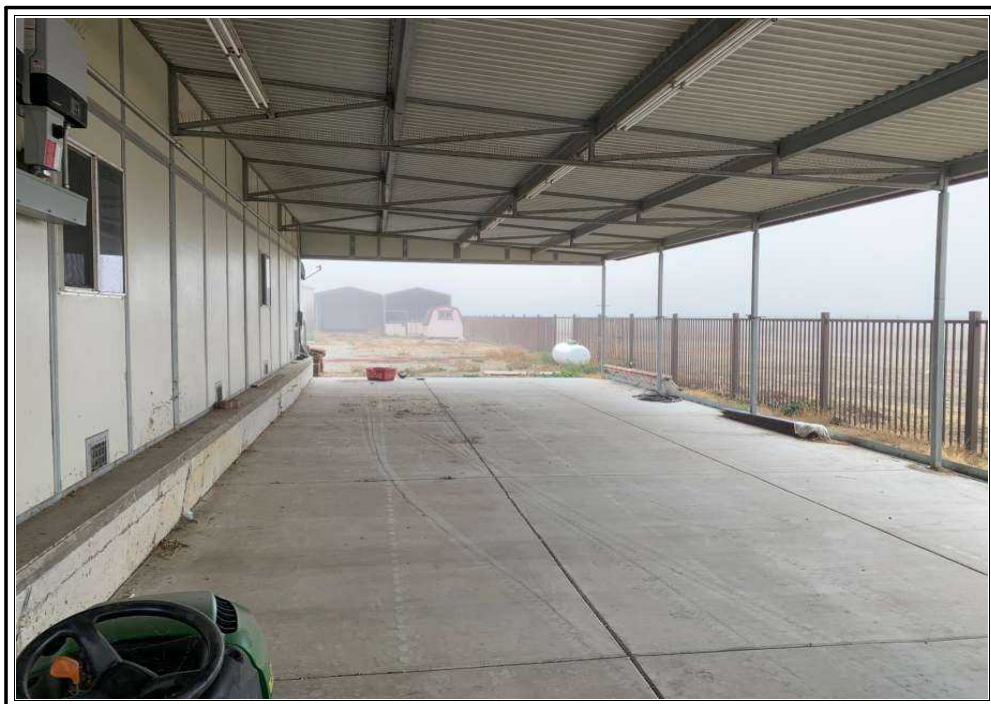
Covered area of shop 2
