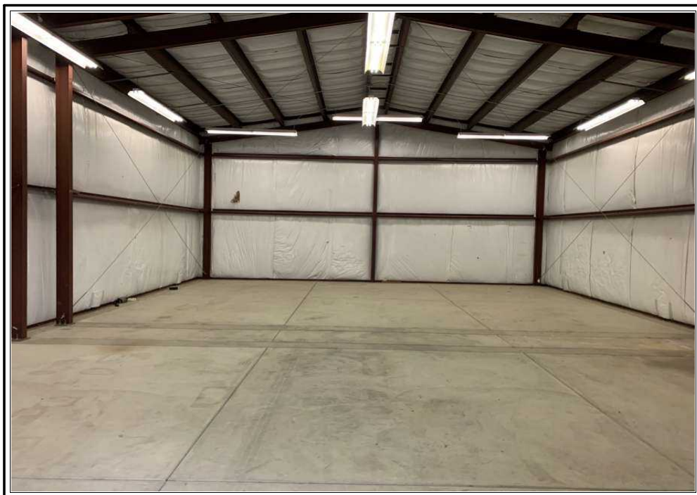
Interior view of shop 1
