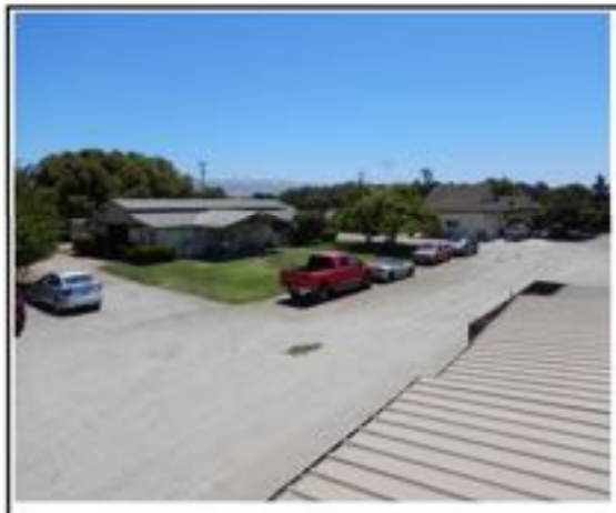
VIEW - HOUSE & BARN
