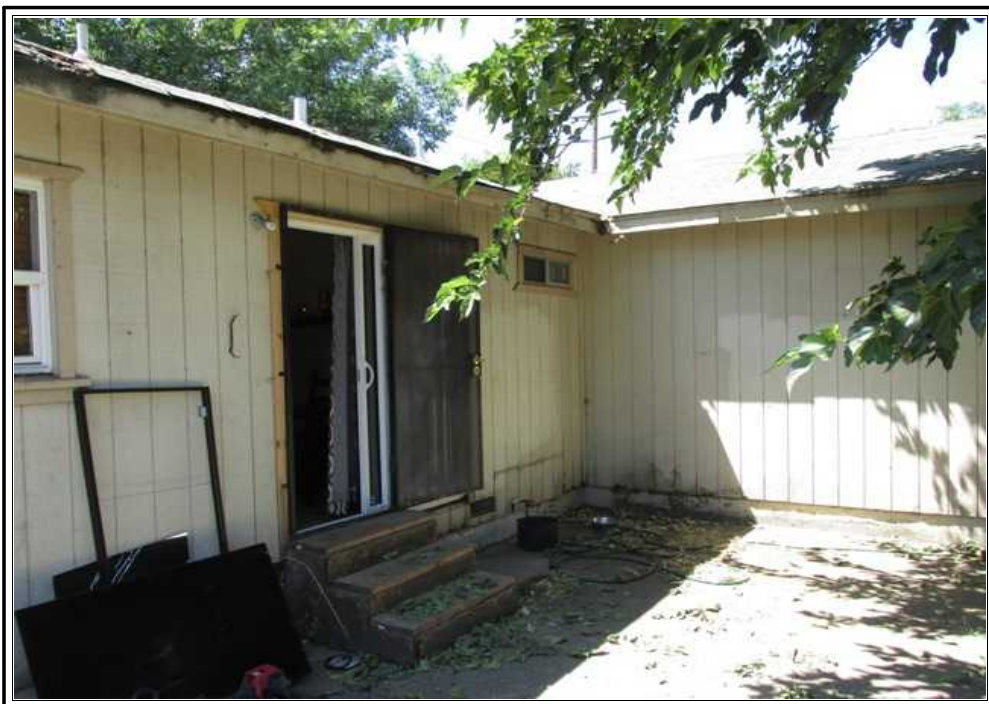
REAR OF SUBJECT PROPERTY
