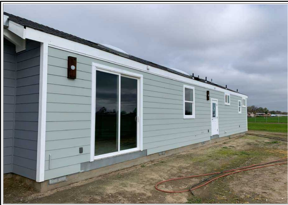
REAR OF SUBJECT PROPERTY
