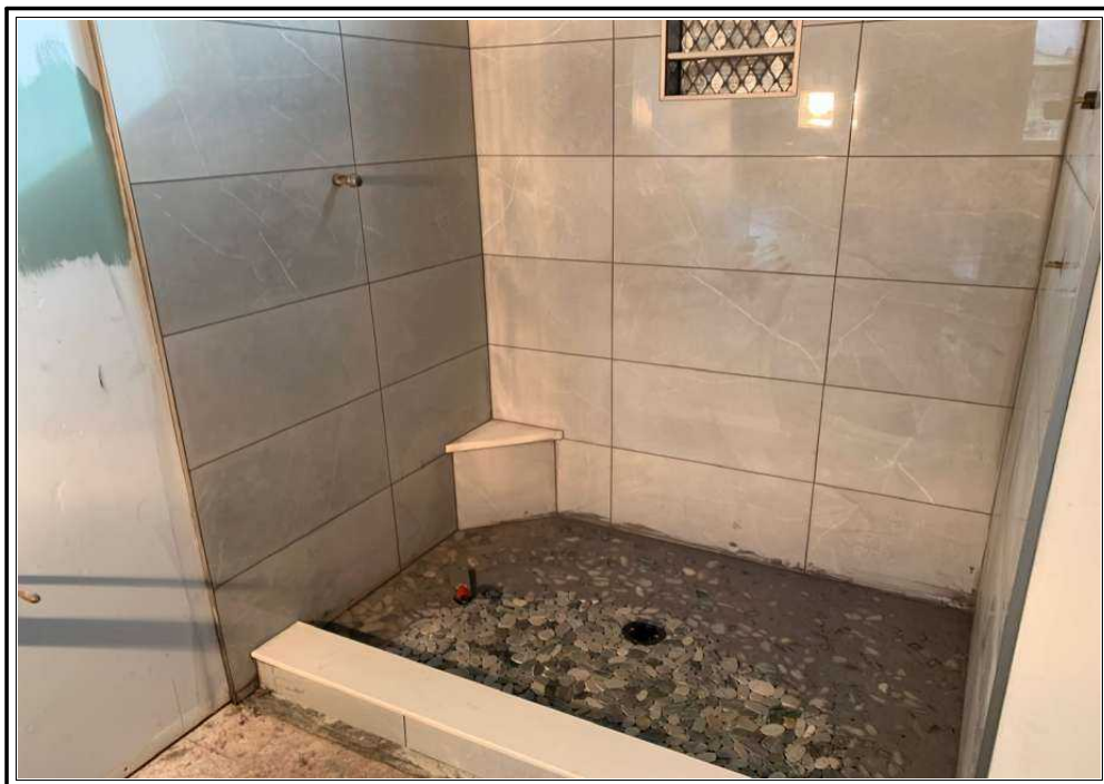
Additional view of Master Bathroom
