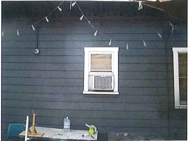
WINDOW AC UNIT
