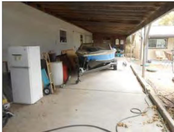
WEST ELEVATION OVERHANG AREA - COMMERCIAL BUILDING
