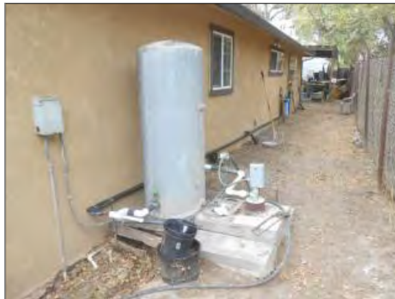
REAR ELEVATION OF SFR WITH PROPERTY DOMESTIC WELL IN FOREGROUND
