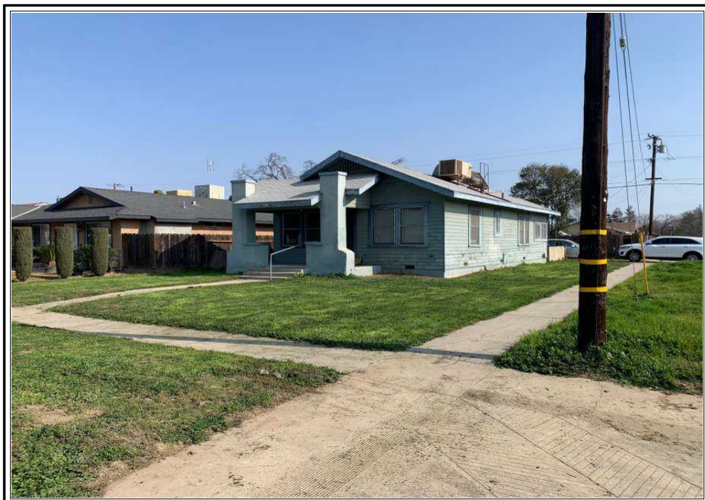
View of subject's corner location
