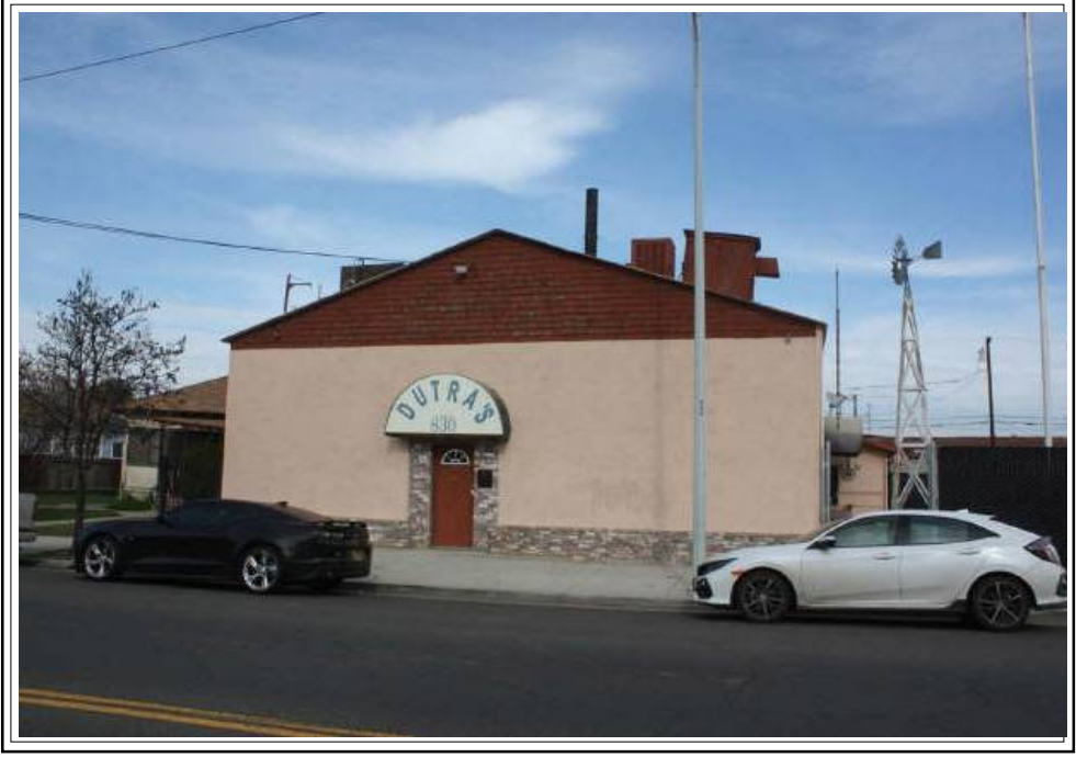
FRONT VIEW OF SUBJECT PROPERTY
