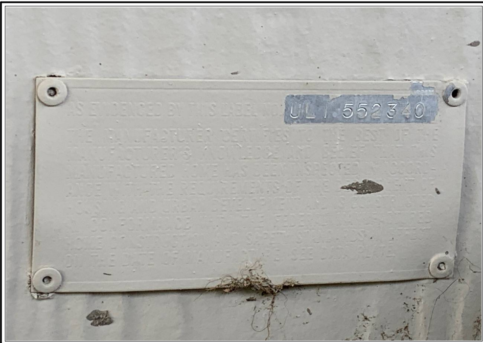
HUD data tag on exterior of Unit 14414
