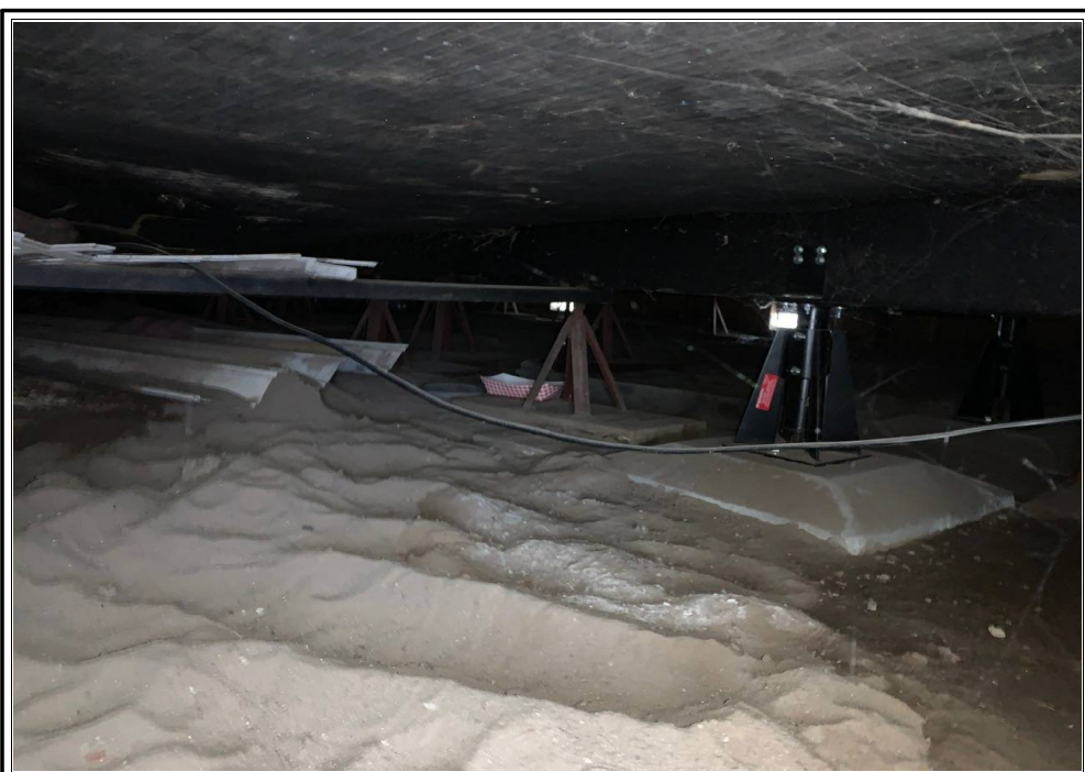
Concrete pier and jack stands foundation
