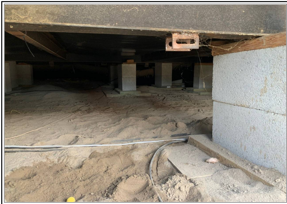
Concrete Block foundation
