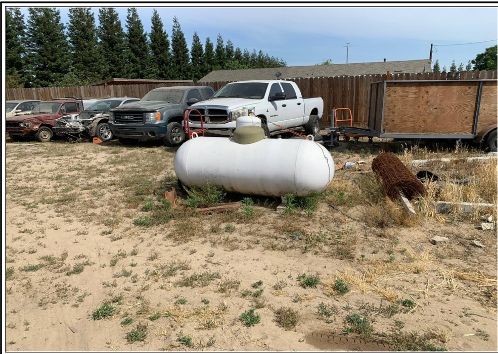
Propane tank for unit 14414
