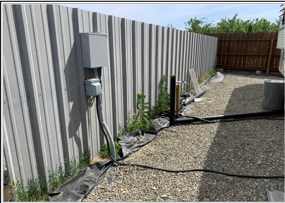
Electrical to site of RV parking
