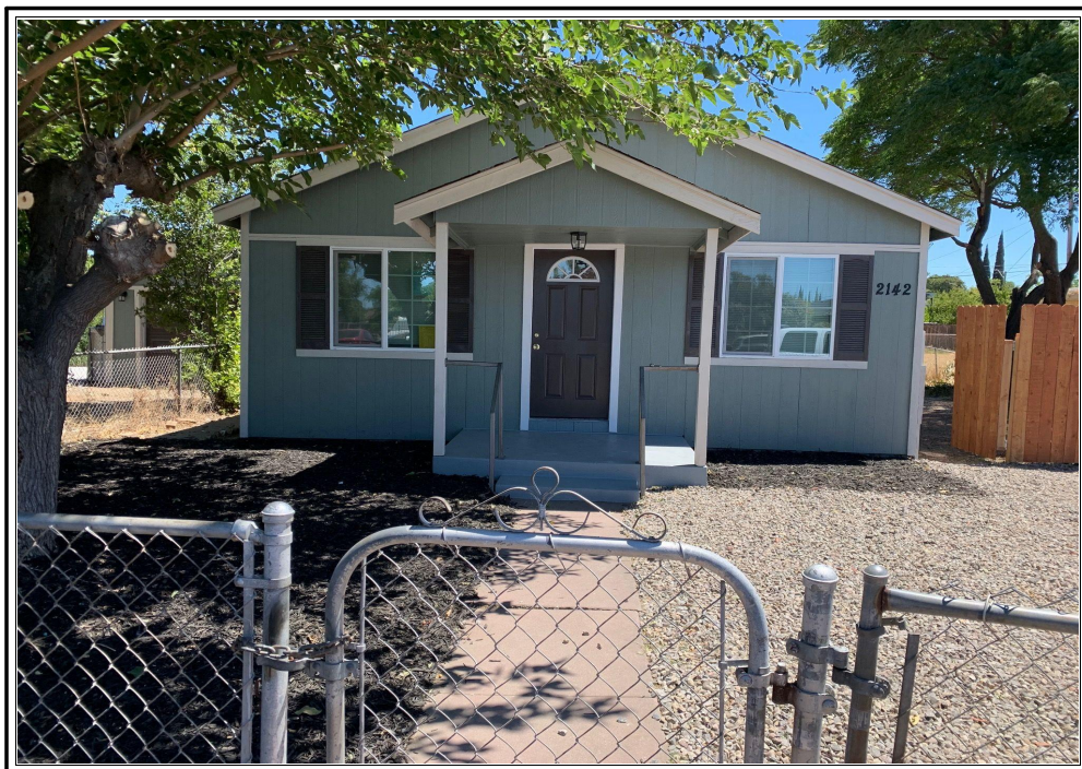
Additional front view of subject
