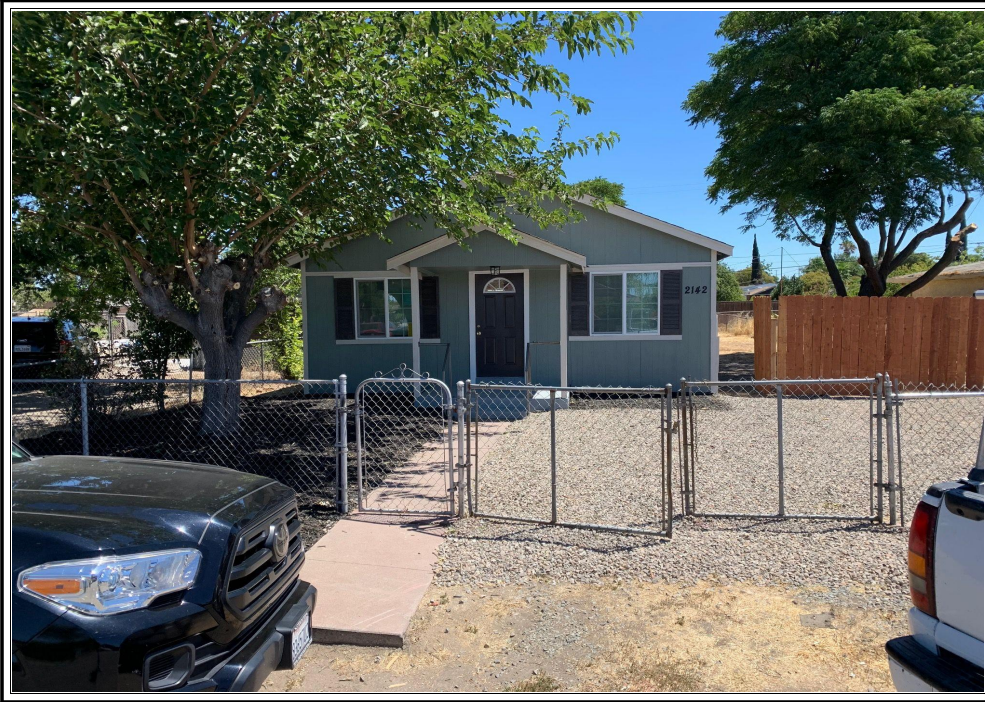
FRONT OF SUBJECT PROPERTY 2142 S Laurel Street Stockton, CA 95206-2436
