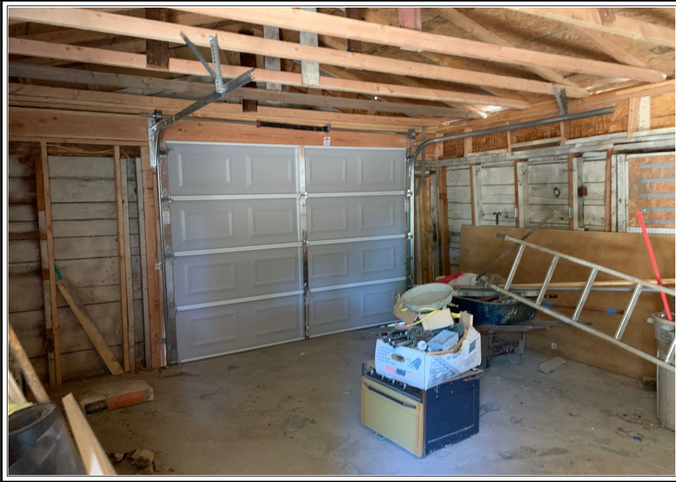
Interior view of Garage
