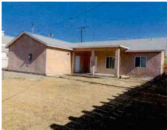
Rear view of subject residence
