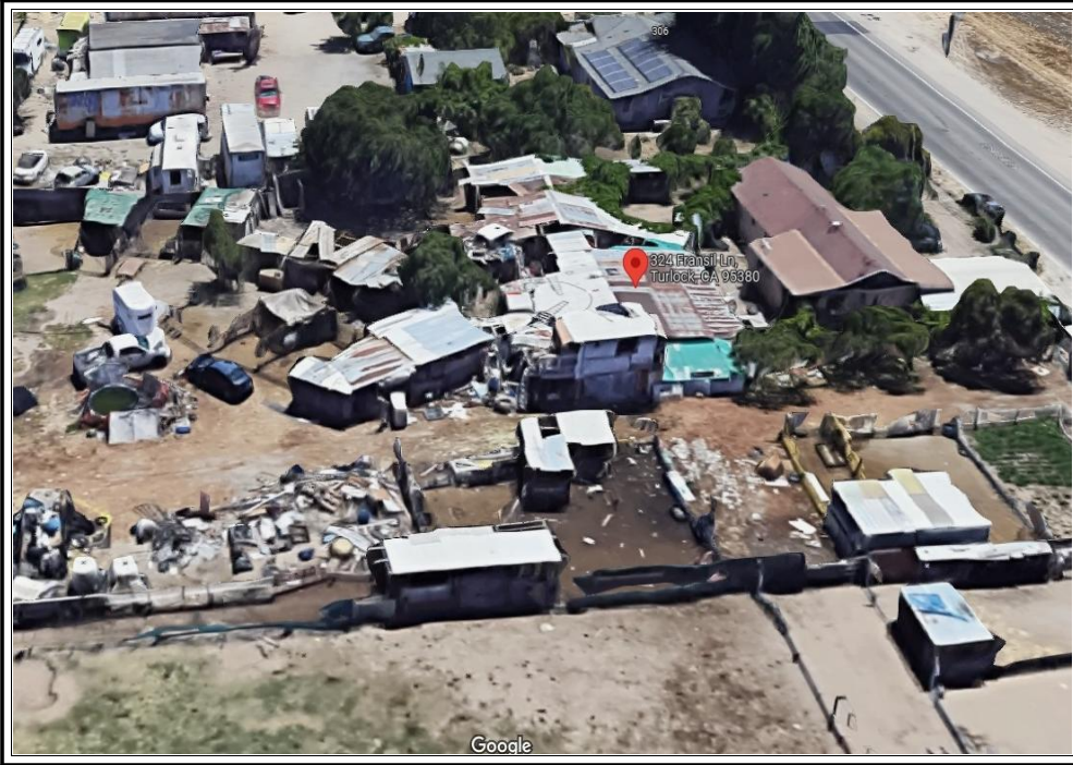
Google Aerial photo of structure to rear of subject
