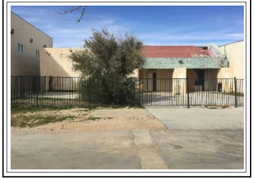
Rear of Building
