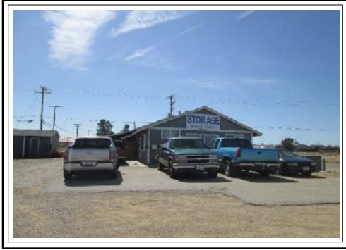
Front Entrance to Subject
