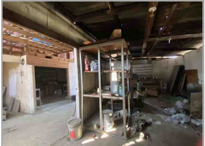
SUBJECT BARN AREA
