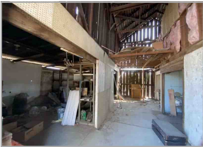
SUBJECT BARN AREA
