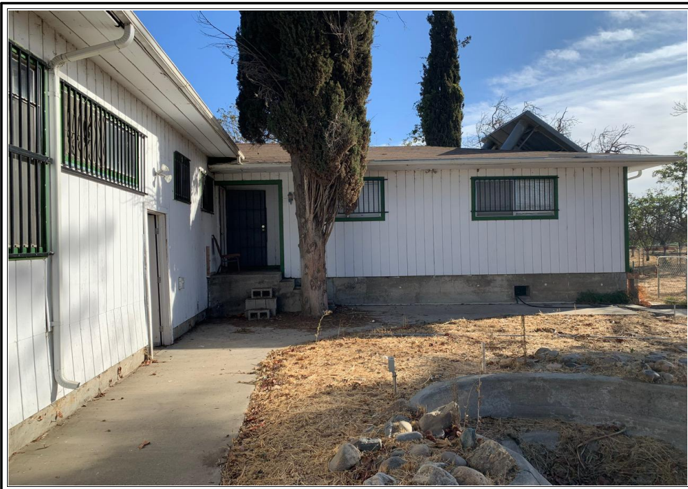
REAR OF SUBJECT PROPERTY
