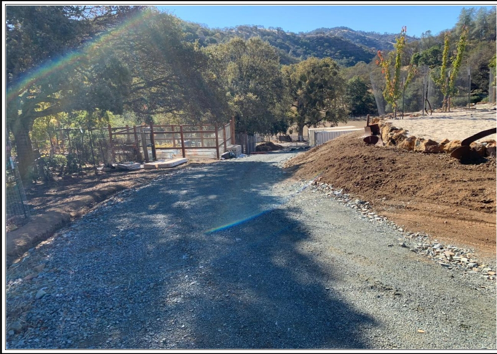
Additional view of gravel driveway
