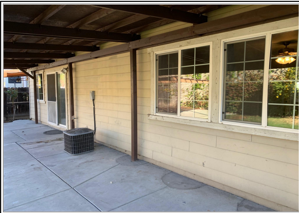
REAR OF SUBJECT PROPERTY
