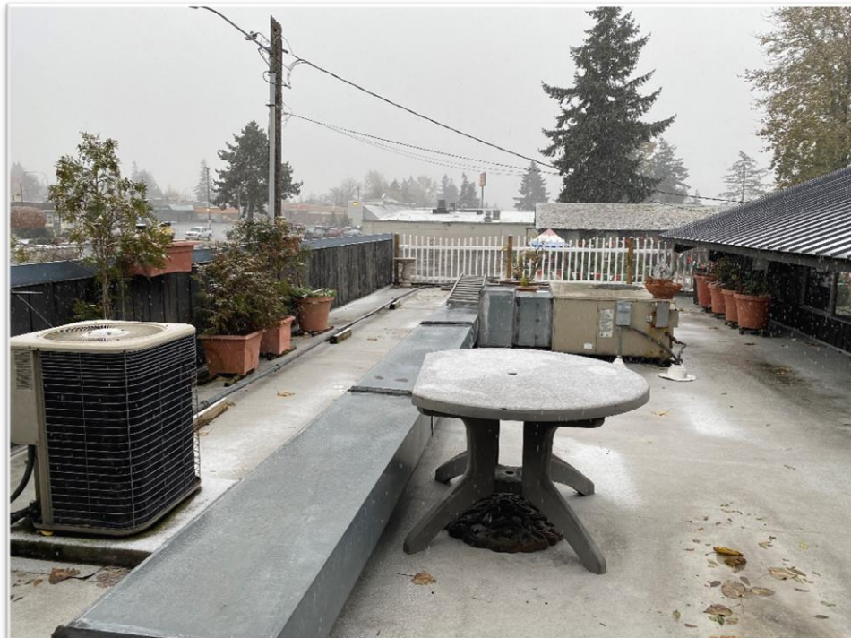
Subject Property Apartment Unit, Deck
