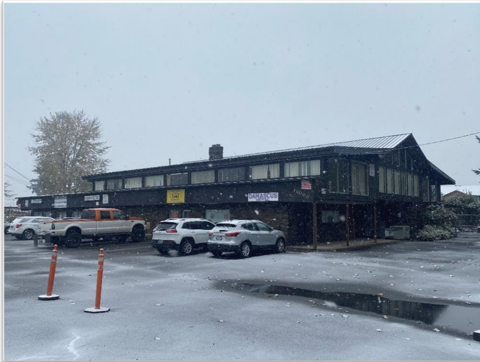
Subject Property North and East Elevations
