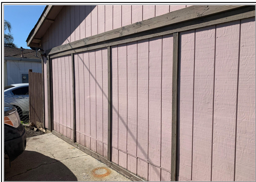
Front view showing garage door has been sealed due to conversion
