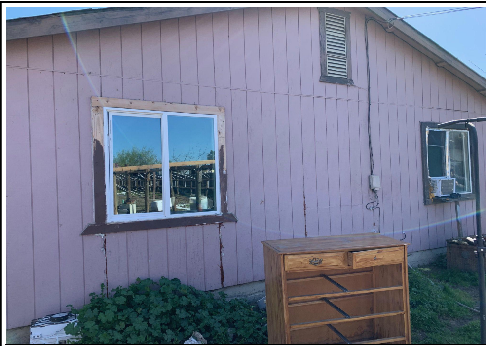
REAR OF SUBJECT PROPERTY
