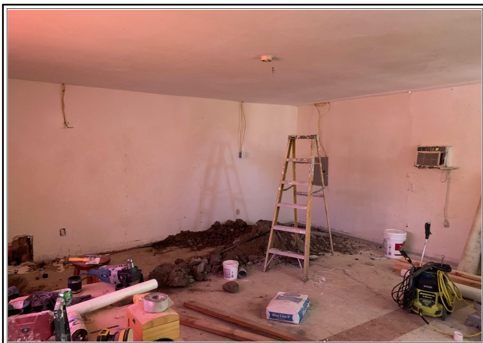
Interior view of converted garage
