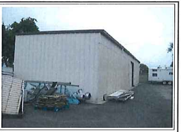
Enclosed Storage Building
