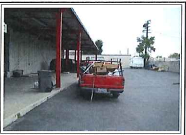
South Side of Warehouse and Asphalt Storage Area
