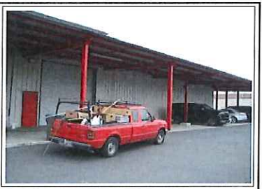
South Side of Warehouse
