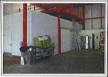
Exterior Cold box
