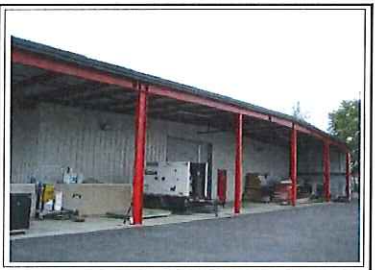
East Side of Warehouse
