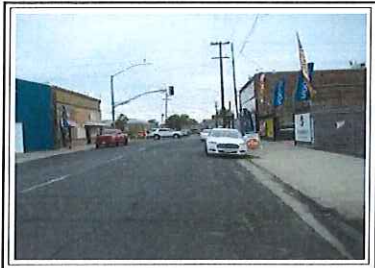
Main Street Looking East
