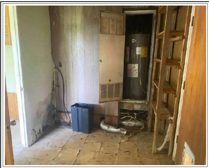
Laundry area Bonus Room
