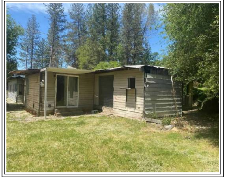
Exterior view of additional rooms and decking
