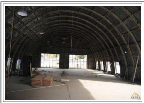
Interior Quonset Building
