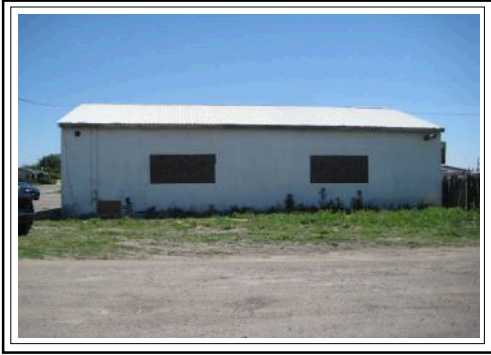
East View of Subject Building
