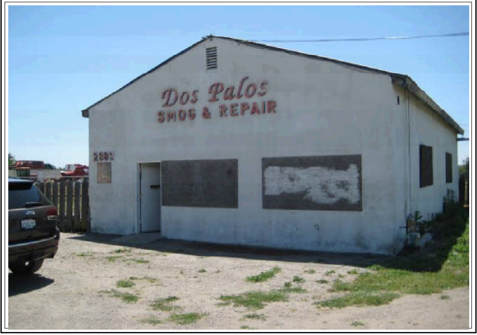
FRONT VIEW OF SUBJECT PROPERTY
