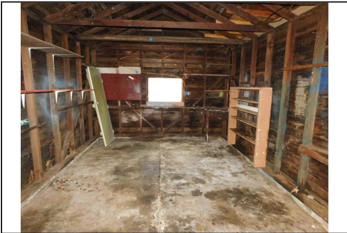
Interior view of the subject single stall attached garage
