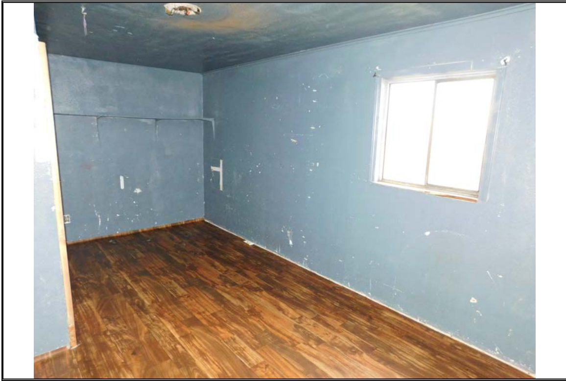
Interior view of the subject dwelling back bedroom
