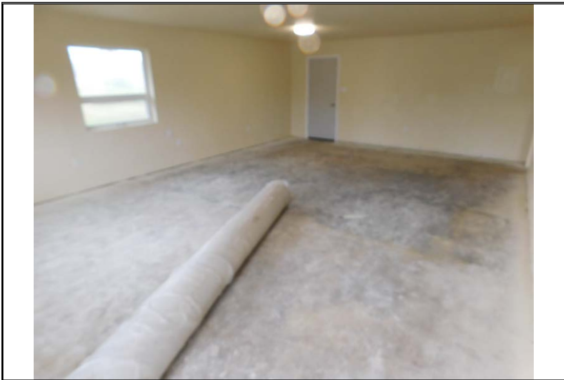
Interior view of the subject office south room with carpet roll to soon be installed
