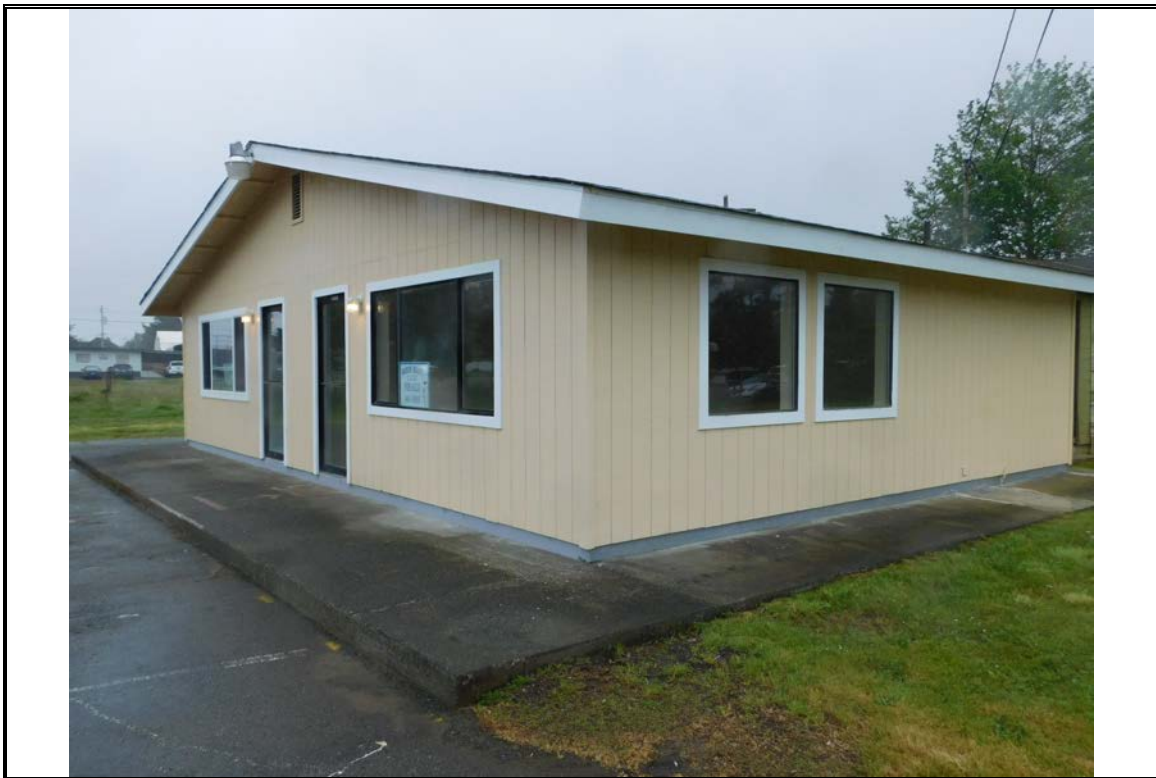
View of the east and north sides of the subject office
