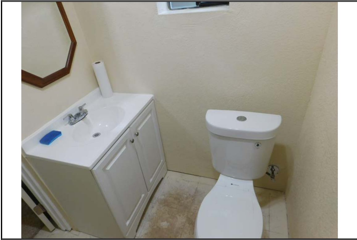
Interior view of the one subject office building restroom
