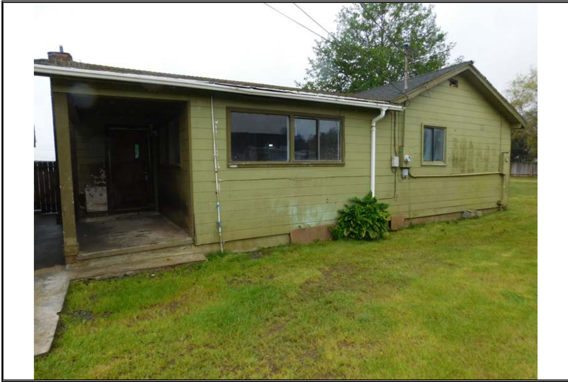
North side view of the subject 2/1 dwelling
