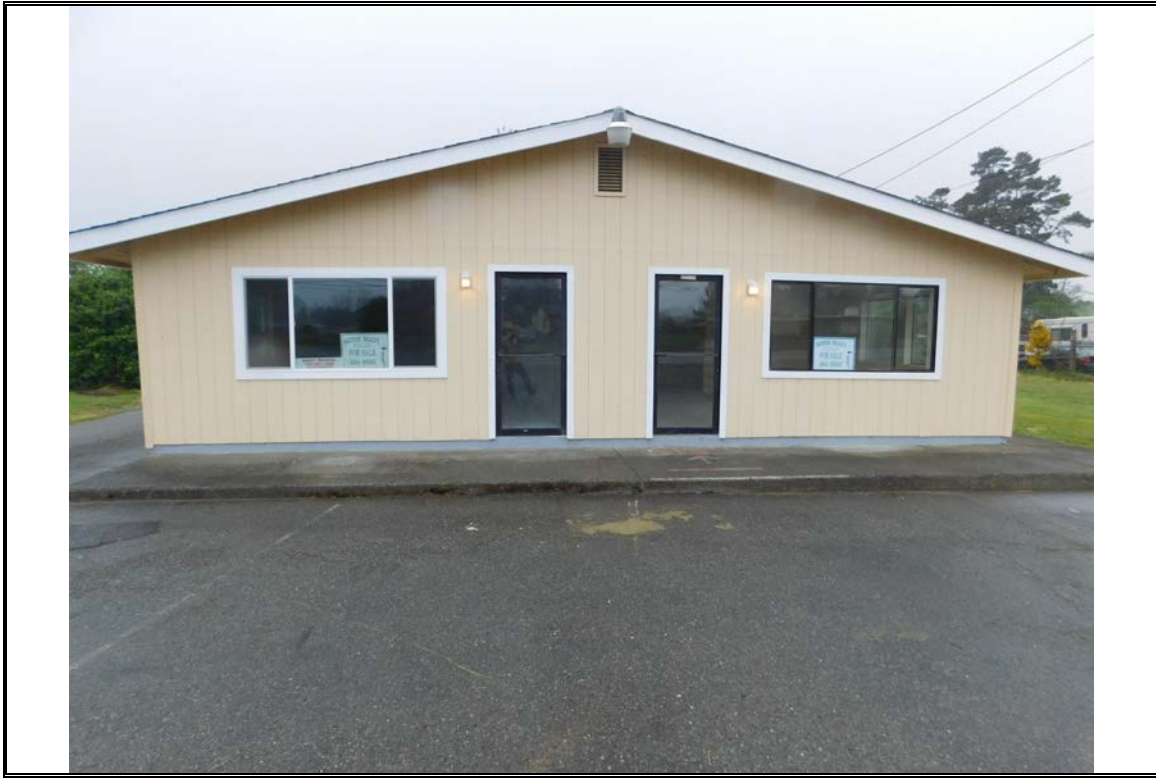
Looking west at the east (front) side of the subject office structure
