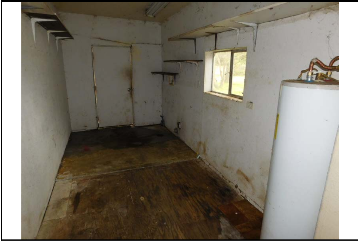
Interior view of subject dwelling laundry room
