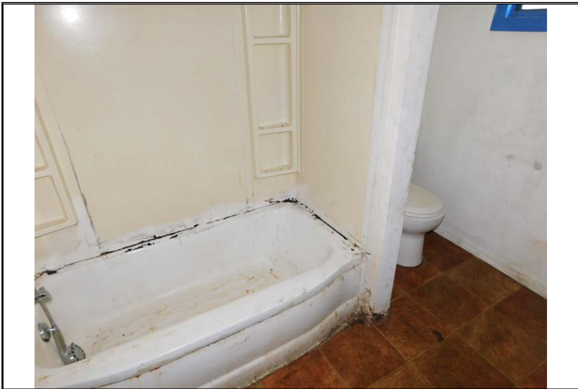
Interior view of the subject dwelling bath
