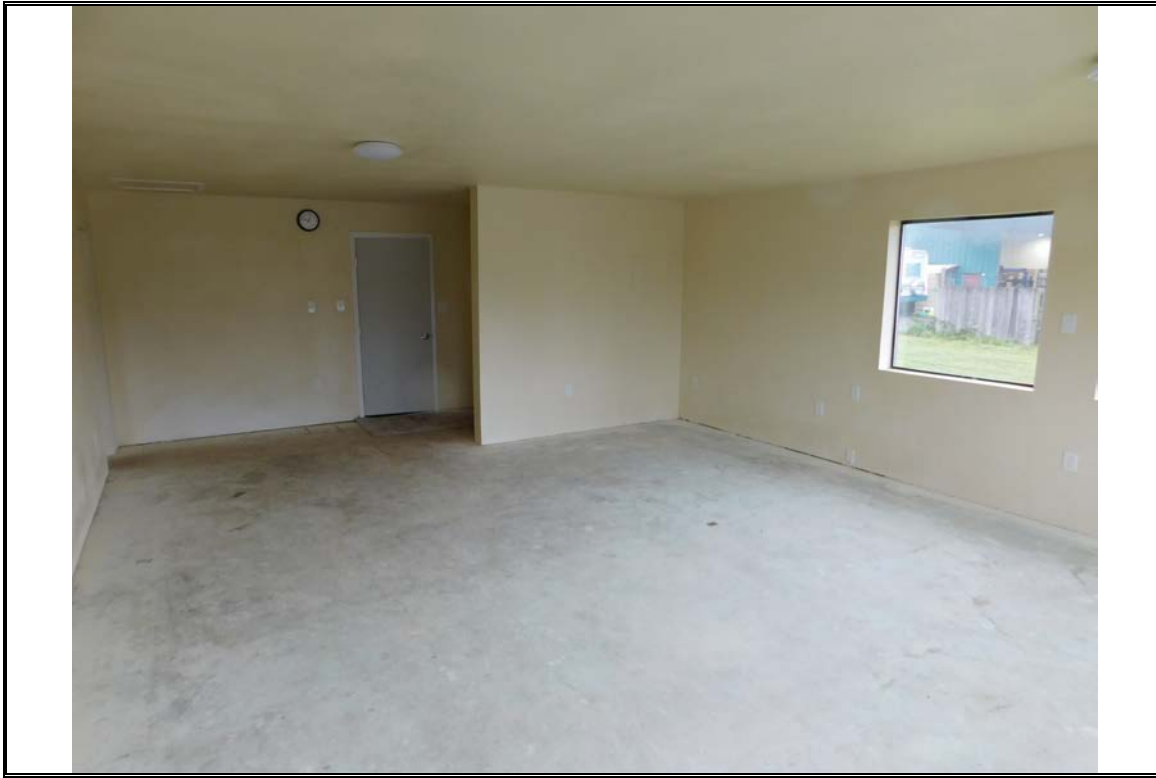
Interior view of the north room of the subject office
