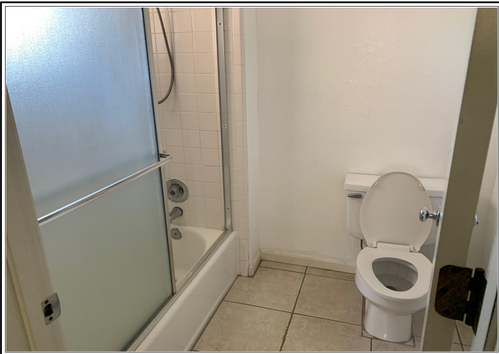
Additional view of Bathroom
