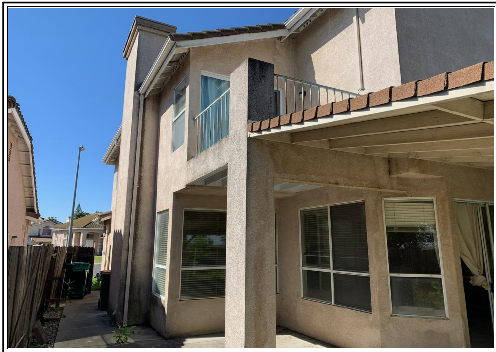
Additional side and rear view of subject
