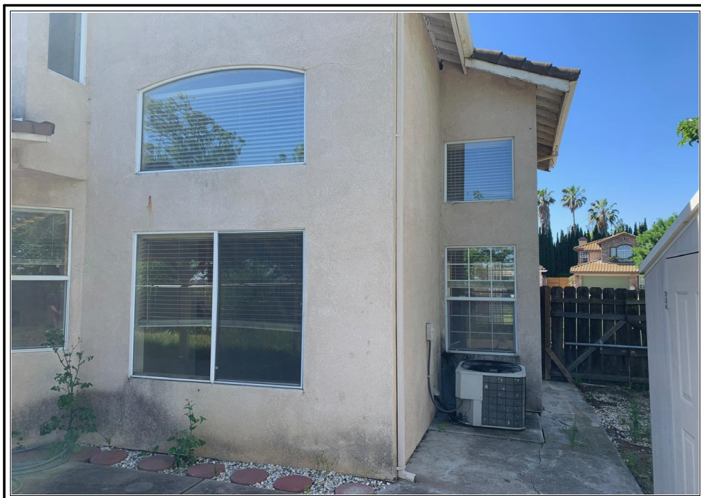
Additional side and rear view of subject
