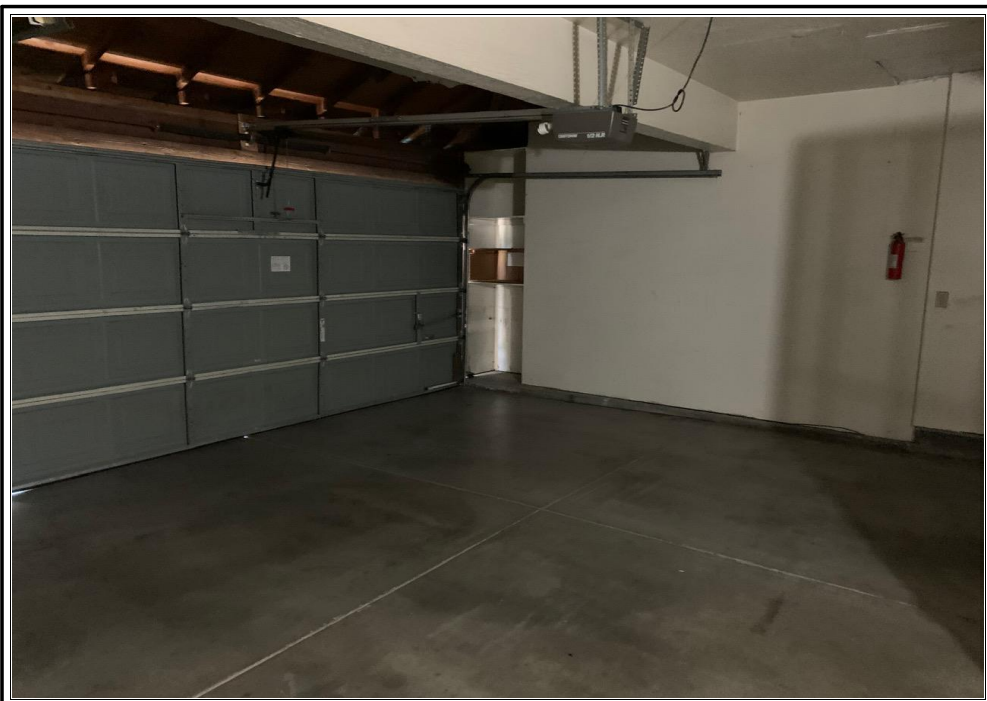
Interior view of Garage
