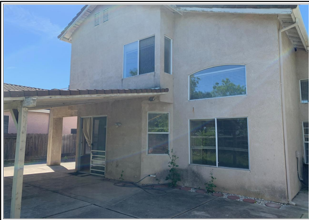
REAR OF SUBJECT PROPERTY
