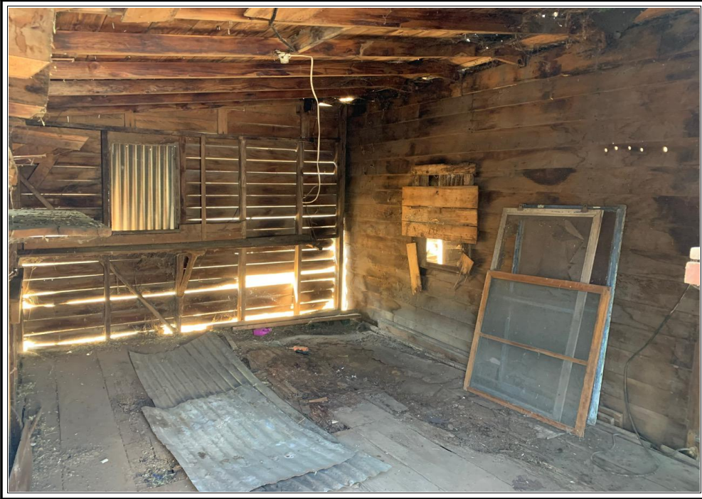
Interior view of shop/storage building
