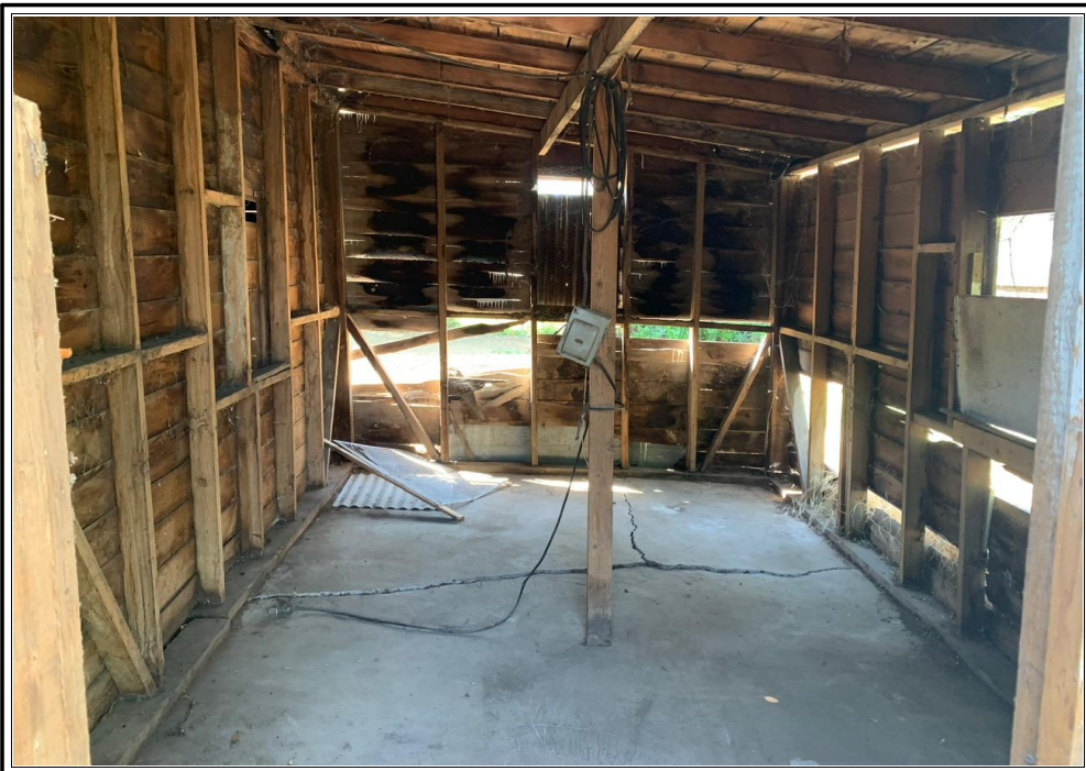
Additional view of shop/storage building
