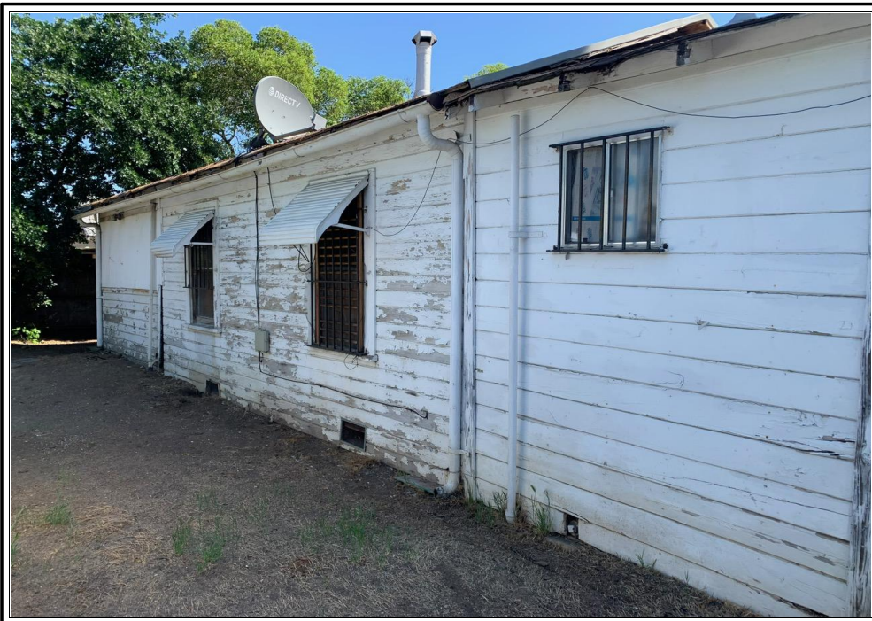
REAR OF SUBJECT PROPERTY
