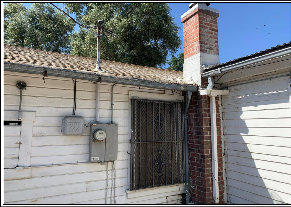
Additional view showing roof
