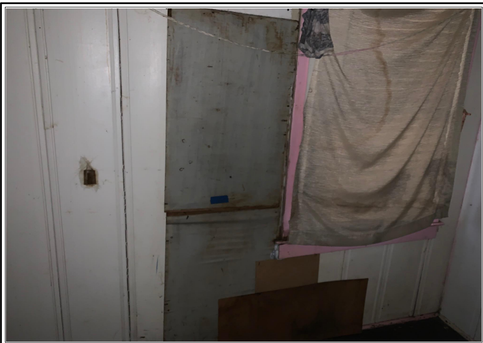
Patched wall in Bedroom
