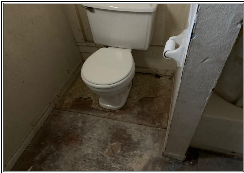
Additional view of Bathroom - showing vinyl floor coverings removed
