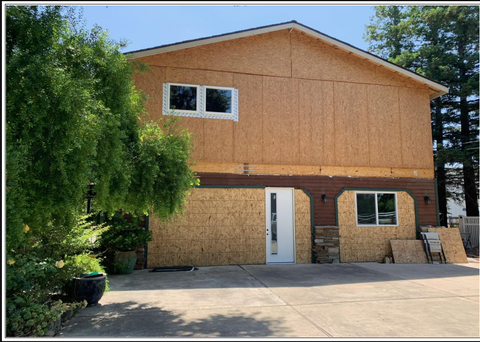
Accessory Dwelling Under Construction
