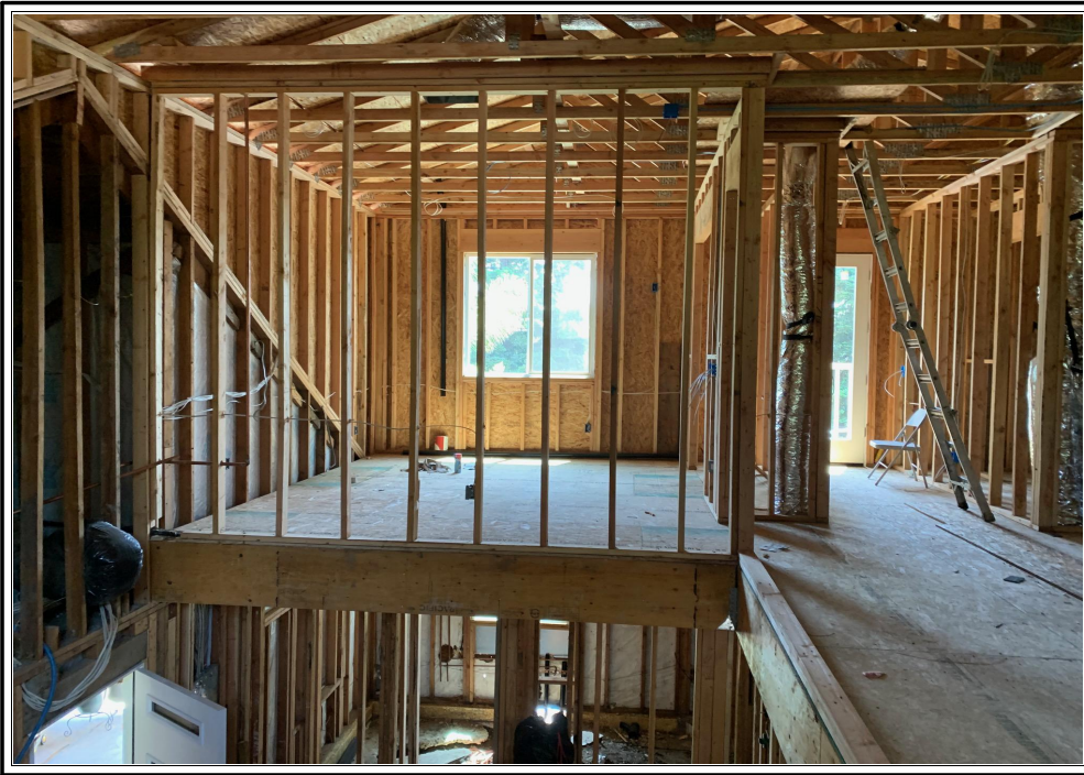
Interior view of Accessory Dwelling Second floor framing complete
