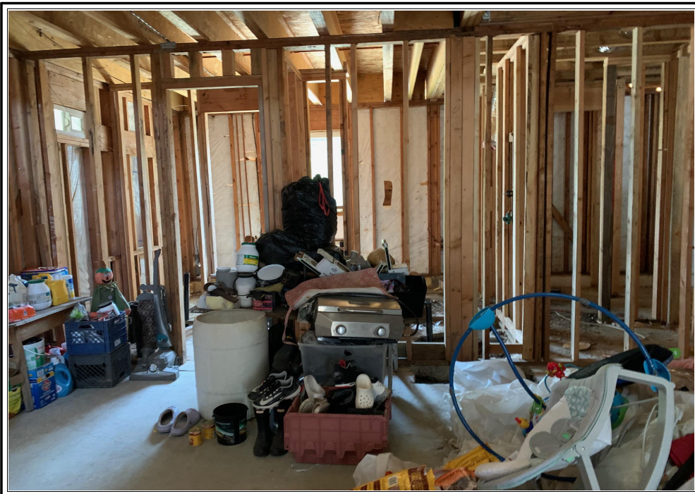
Interior view of Accessory Dwelling Rough framing of interior complete
