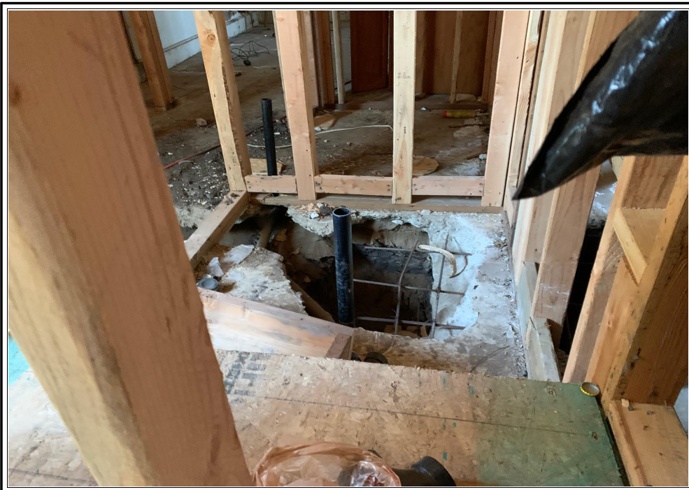
Interior view of Accessory Dwelling Area of removed concrete for plumbing
