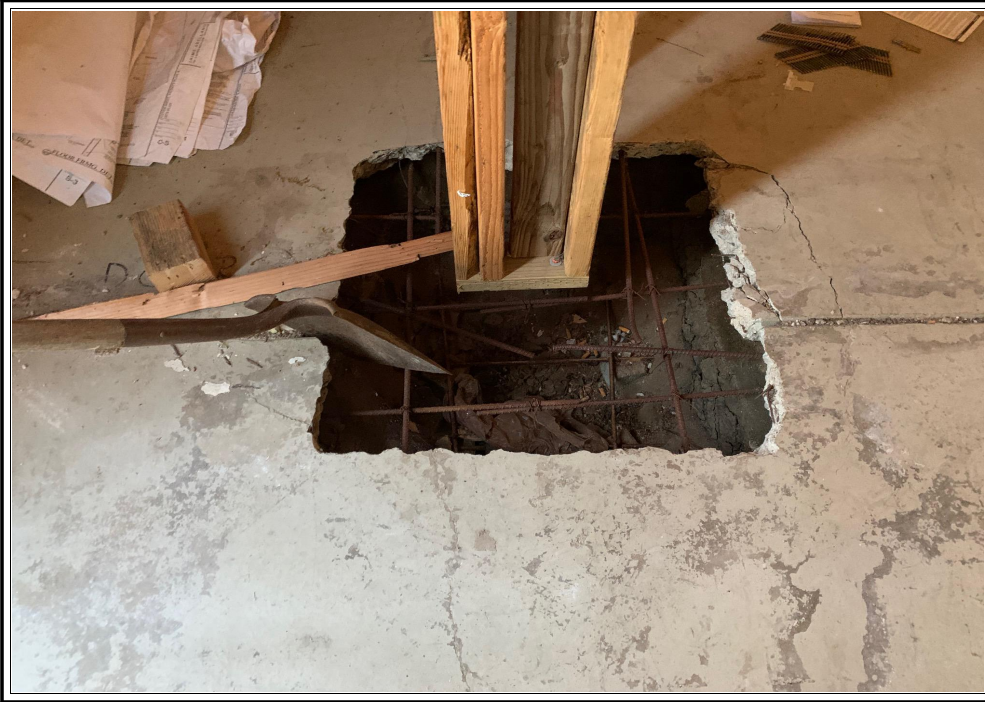
Interior view of Accessory Dwelling Reinforced footing to be poured
