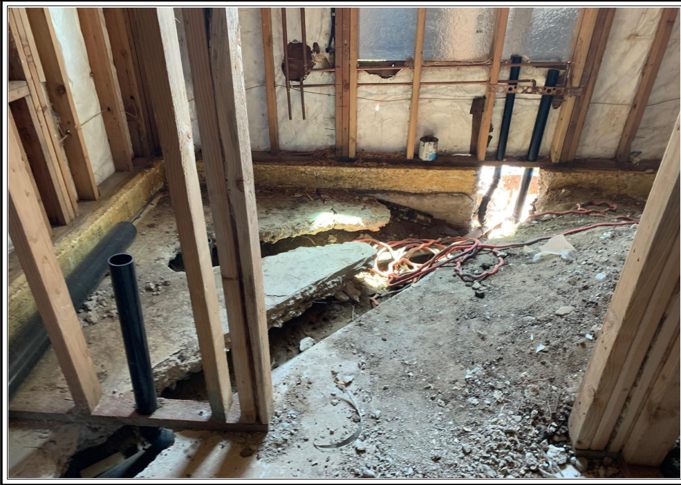
Interior view of Accessory Dwelling Rough plumbing installed
